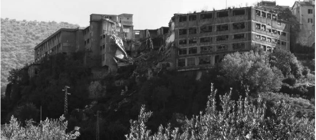
Figure 2. Present day situation: in the image (2020), we can see the actual state caused by the 2009 massive collapse, immediately upstream of a section of “Via degli Stabilimenti” that runs through a tunnel. (from the Technical-illustrative report of the “Design Competition for the construction of the auditorium and car park in the area of the former Amicucci Parmegiani paper mill” - source: Municipality of Tivoli)
