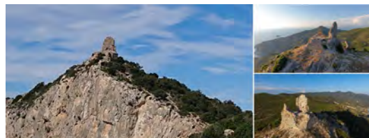
Fig. 1 – Approach to the tower from the south-west crest and aerial views from the south and west.
