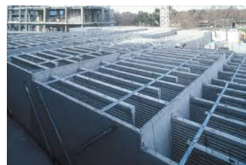
Figura 3.3 Tipologia orizzontale del TLVS presso il Federation Square (Melbourne, Australia). Fonte: Australian Institute of Refrigeration, Air-conditioning and Heating – AIRAH 100 Faces (#042) – Federation Square, Melbourne.
