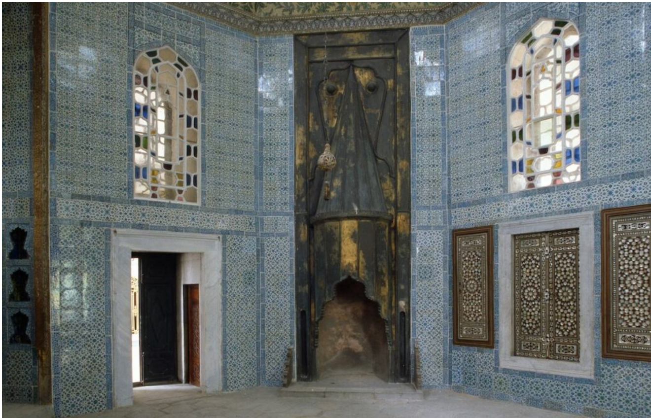
Fig. 1. The metal-sheathed traditional fireplace at the Yerevan Kiosk ( Revan Köşkü , 1635). Topkapı Palace, Istanbul. © Image courtesy of Aras Neftçi.
