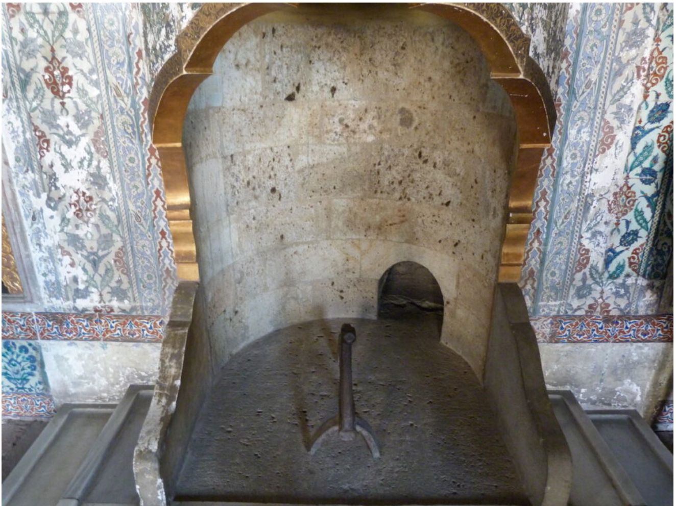
Fig. 4. The firebox of Osman II’s privy chamber (c. 1621). Topkapı Palace, Istanbul. © Derzsi Elekes Andor. Image in the public domain. Image Source: Wikimedia commons .
