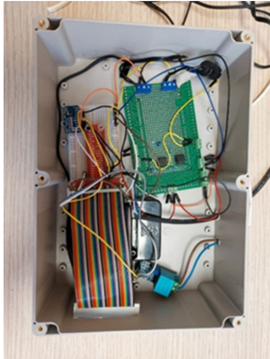
Figure 46: The prototype system set-up in the outdoor box
