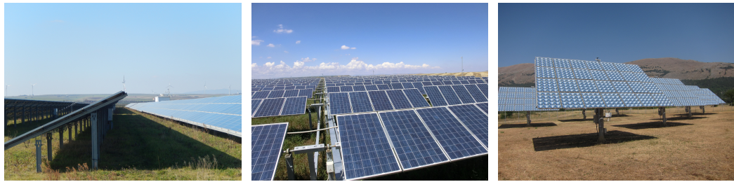
(a) Zimmermann tilted-fixed systems (b) Convert flat uniaxial tracking systems (c) Solfocus biaxial tracking systems with high-concentration photovoltaics
