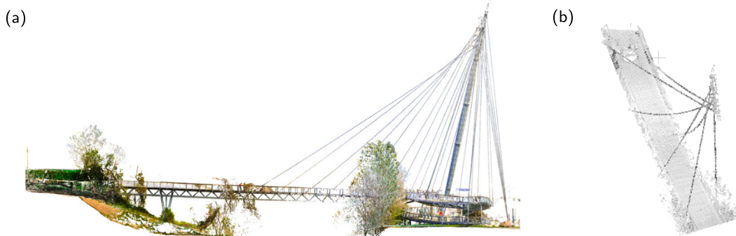
Fig. 6. Point cloud model of the Albano Zuin bridge: (a) lateral view of the complete color point cloud model; (b) aerial view of the model region including the seven stay cables supporting the deck.
