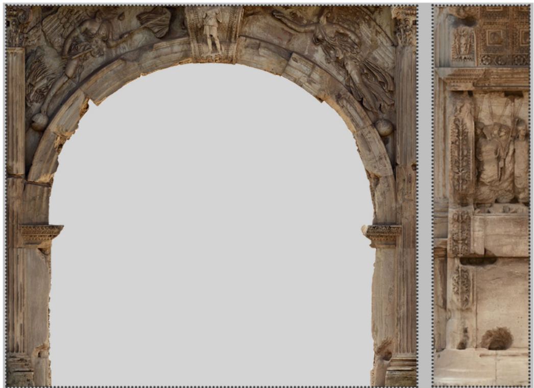
Fig. 7. Gigapixel orthophoto of the Arch of Titus. On the left the detail of the cornice of the fornic; on the right the intrados of the arch with the decoration of the pilasters and the impost capital. Authors' elaboration.
