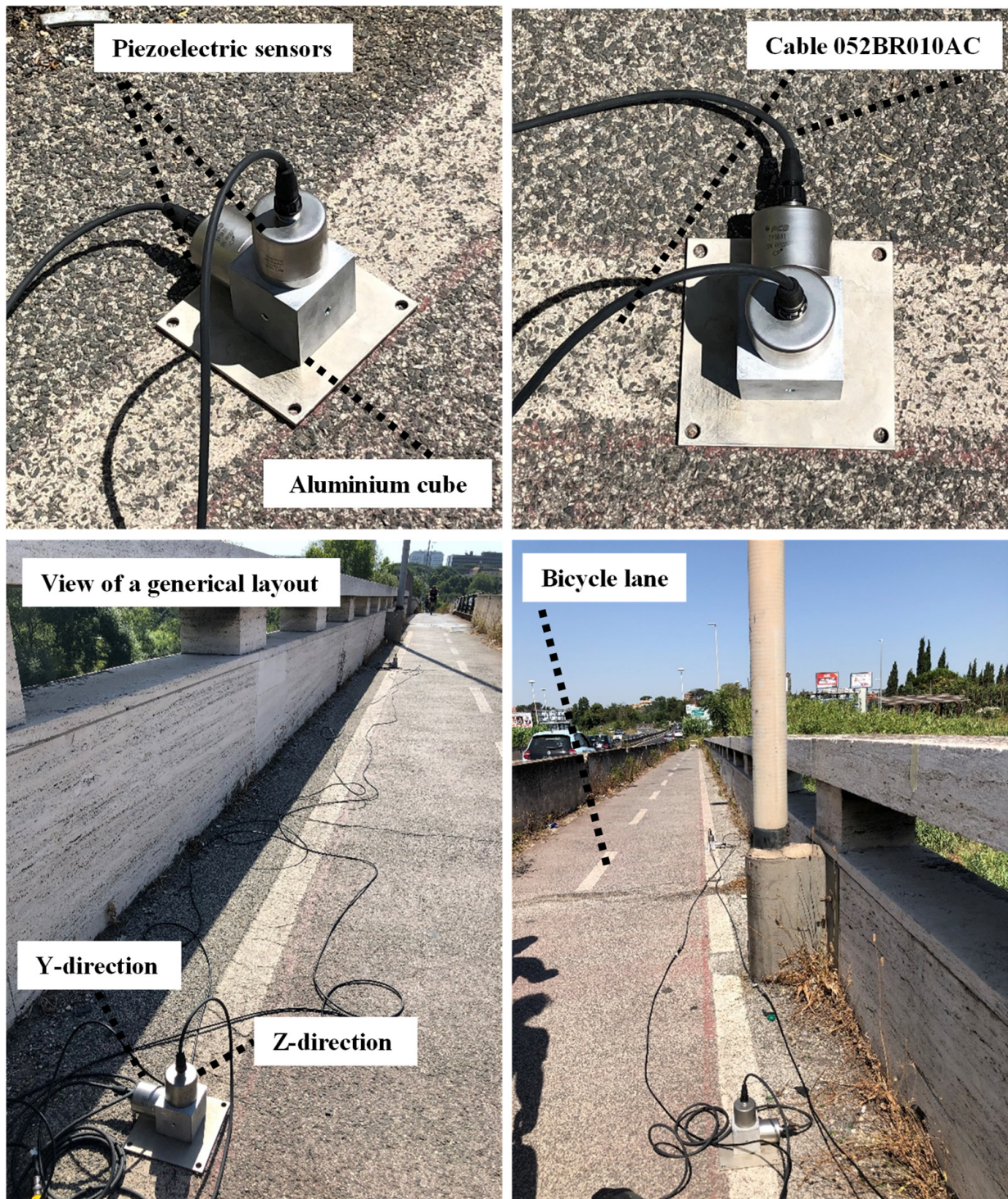
Figure 6. Accelerometers and examples of the experimental layout installation on the bridge.
