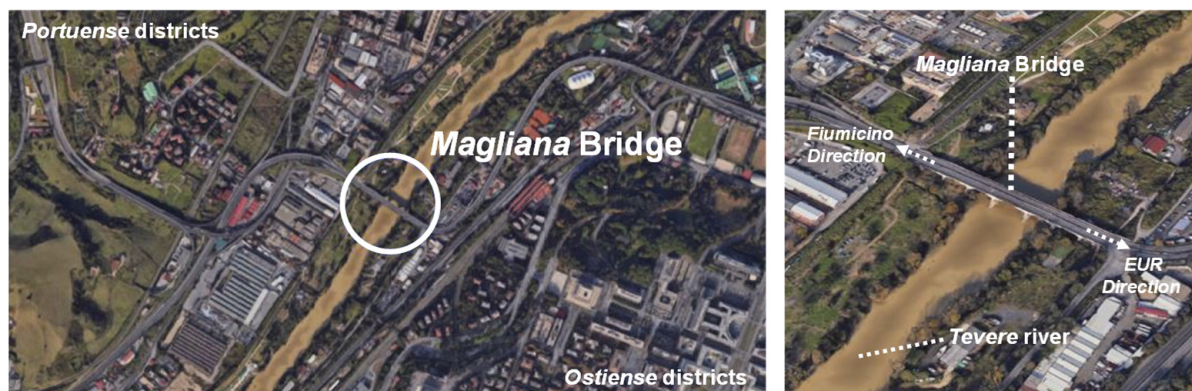
Figure 3. Overview and zoom of the "Ponte della Magliana" bridge in the urban context.
