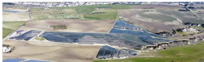
Fig. 1. Aerial view of the Ferrandina plant.
