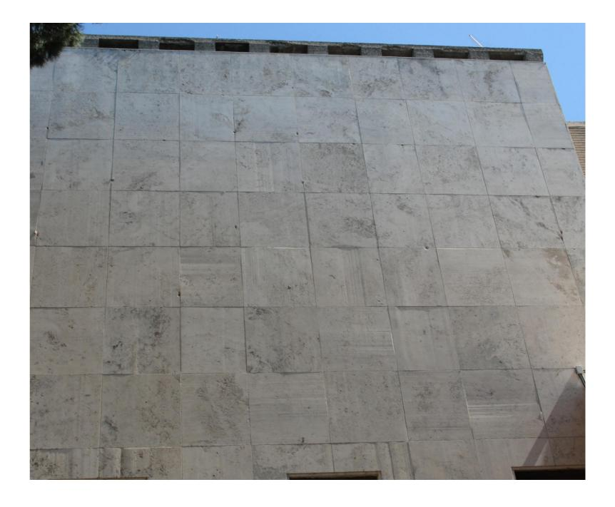
Figure 14 - The travertine cladding on the southwest elevation photographed with sidelight in order to show the degradation of the slabs (© Salvo 2020)
