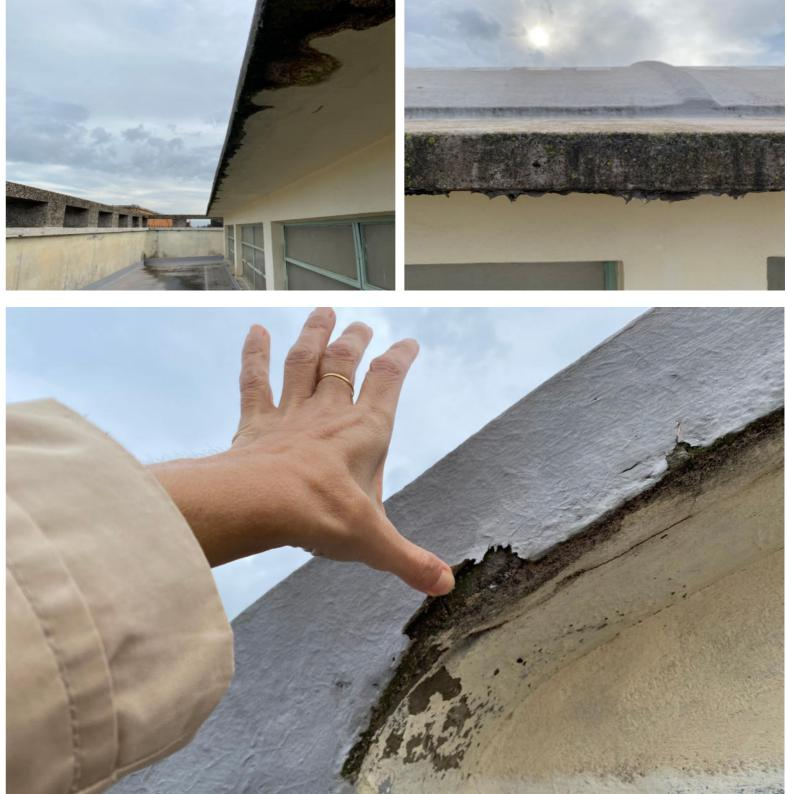
Figure 15 a/b - The condition of the fiber-reinforced resin coating applied in 2013 on the roof and skylights of the library (© Salvo 2021)
