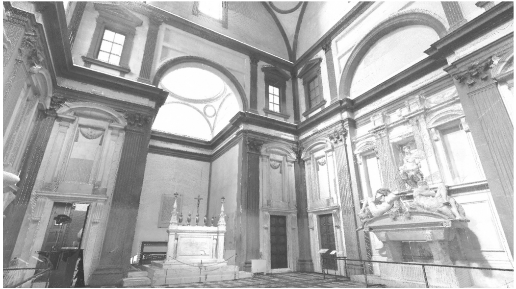
Fig. 3. Internal view of the Sagrestia Nuova. 3D point cloud.
