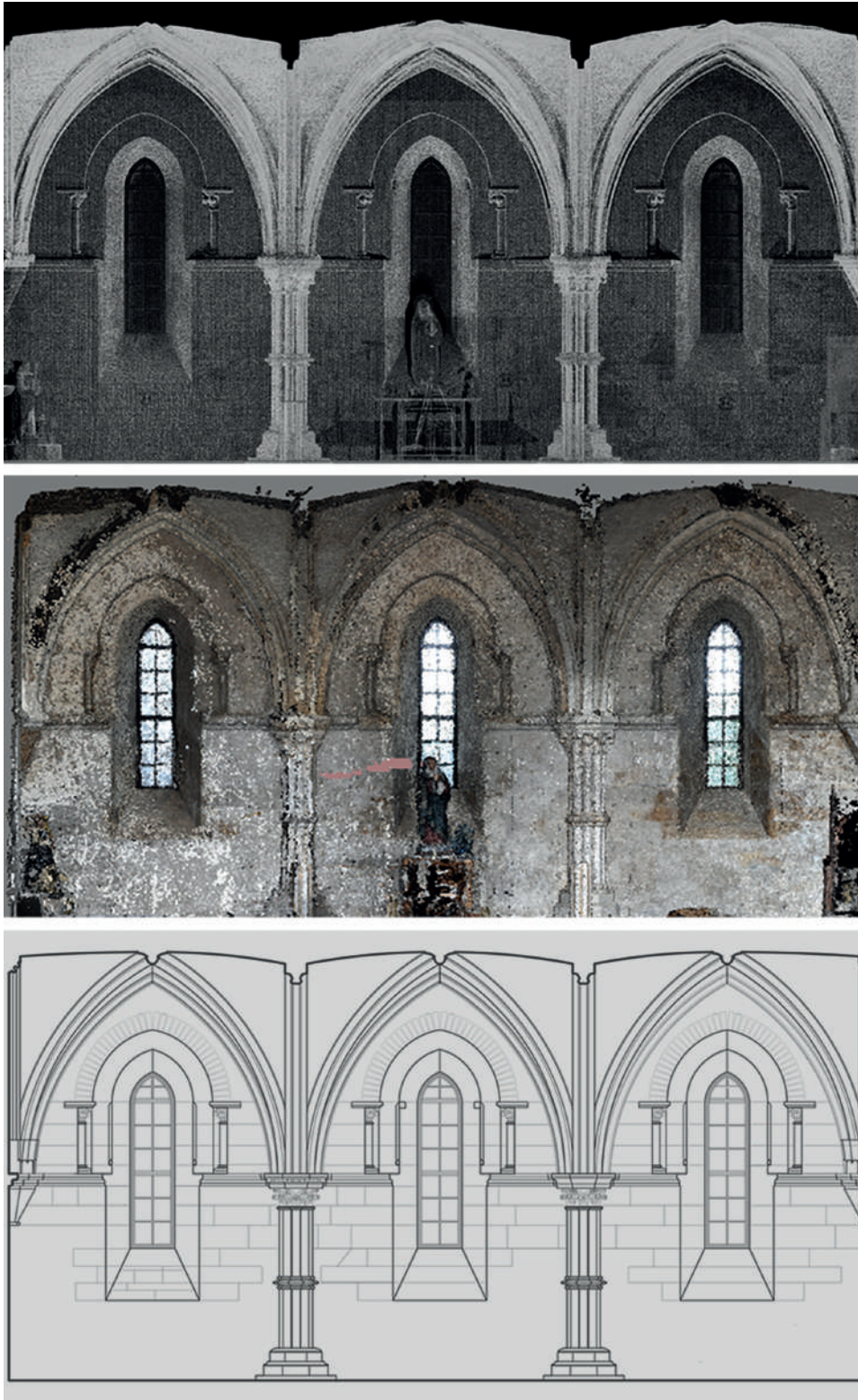
Figure 6. Architectural scale, the Chapter House: numerical model derived from laser scanning, numerical model derived from Structure from Motion and Image Matching, architectural 2D model.
