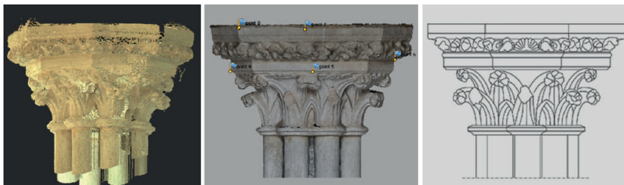
Figure 7. Detail scale, the Capital: numerical model derived from laser scanning, numerical model derived from Structure from Motion and Image Matching, architectural 2D model.
