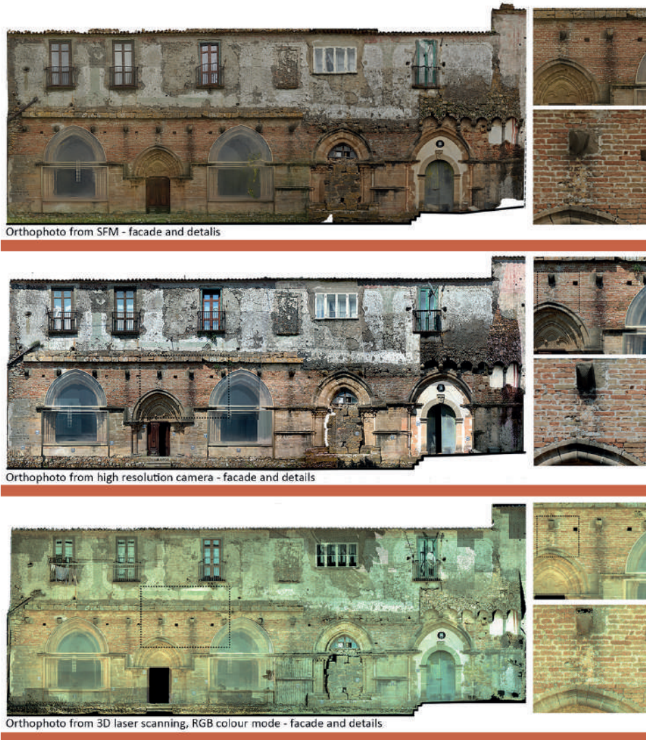
Figure 9. Orthophoto of the façade obtained through three different methodologies: High Resolution camera, Structure from Motion and Image Matching, Laser scanning-RGB mode. Comparison about RGB data.
