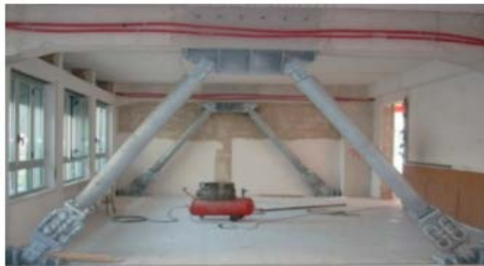
Figure 10. Vibo Valentia school (Italy). Example of a bracing system with HBF.
