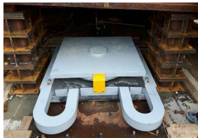
Figure 8. Aurelia-La Rusca Viaduct (Italy). The AIOS consists of elastoplastic elements coupled with spherical bearings due the greater rotations in railway applications.
