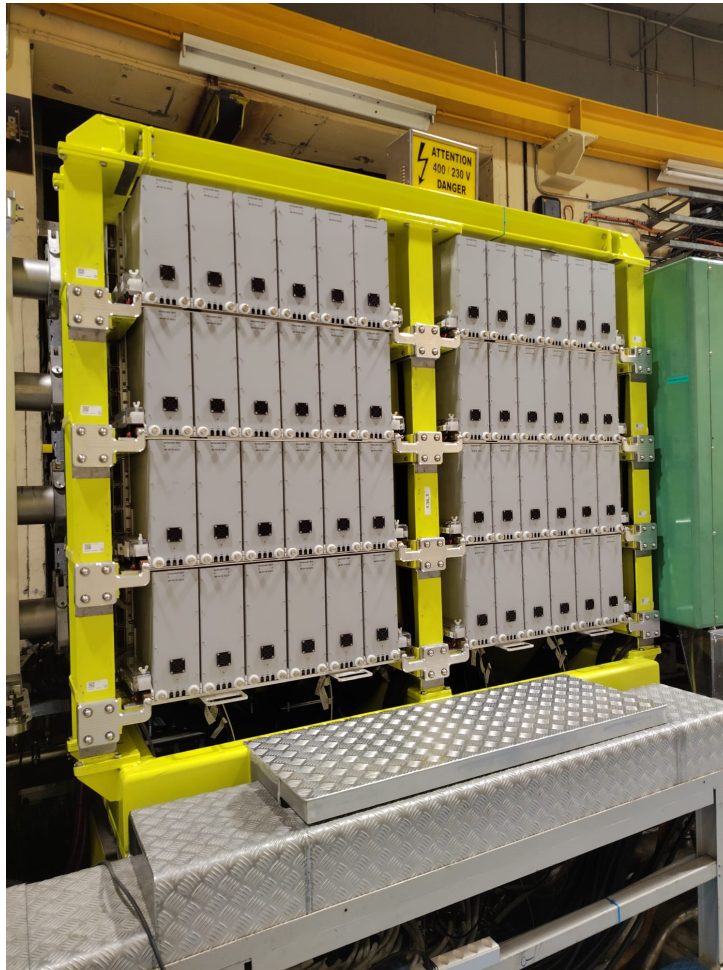
Figure 3.1: One Finemet RF station in a PSB straight section.
