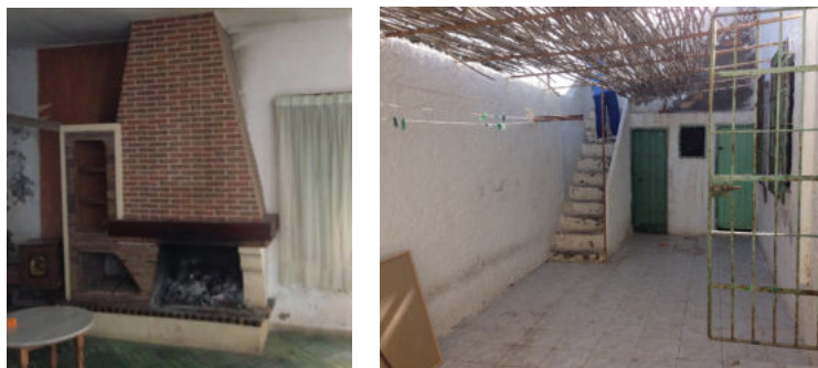
En la Ortila - Prima, Ante Operam, Before renovation
