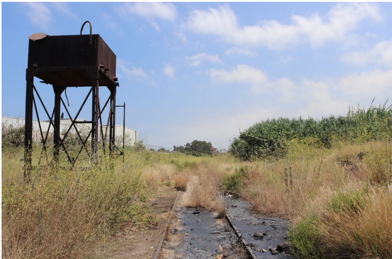
Abandoned water tower and rusting rails define the historical landscape of the complex (photo by Yara Rizk)
