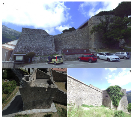
Fig.03. 1. North-east view of the fortress. Notice the difference in height between two bastions and the sloped contour of the connecting that connect them; 2. top view of the watchtower on the west bastion; 3. South-west. south-west view. Notice the scarp shape of cord in the bastion and linear shape in the wall (pictures by the authors).
