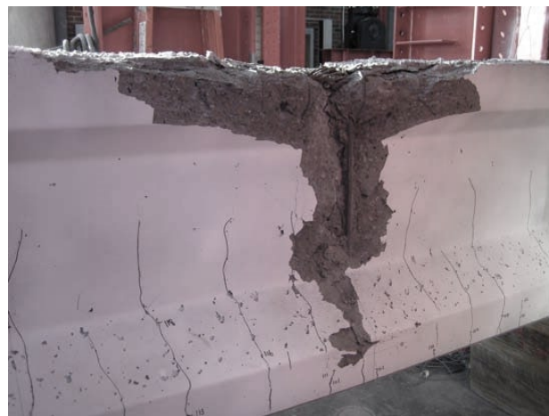
Figure 53: Typical failure modes for the AASHTO girder without deck [105].
