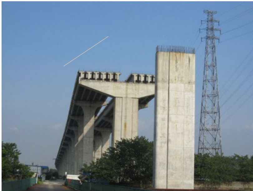
Figure 31: A precast concrete bridge with T-beams [95]
