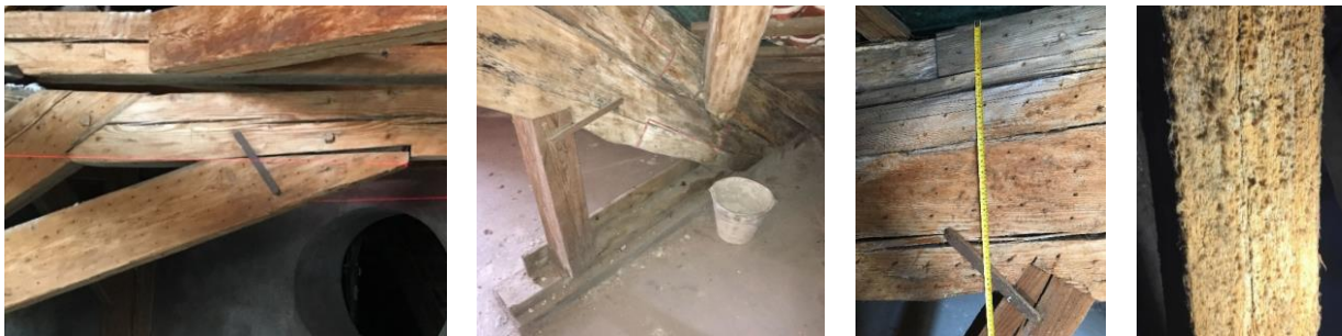
Figure 4 – Characteristic features on the elements from the visual inspection
