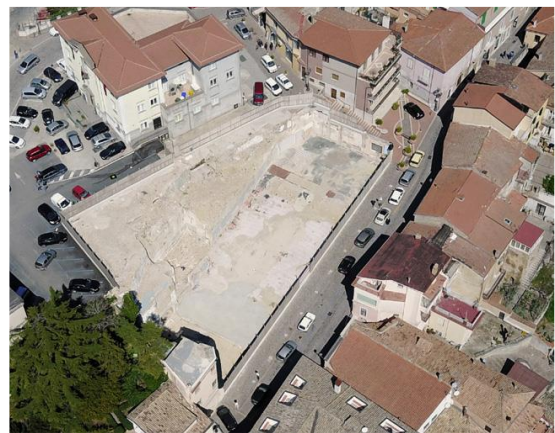
Figure 8. The building site: aerial view
