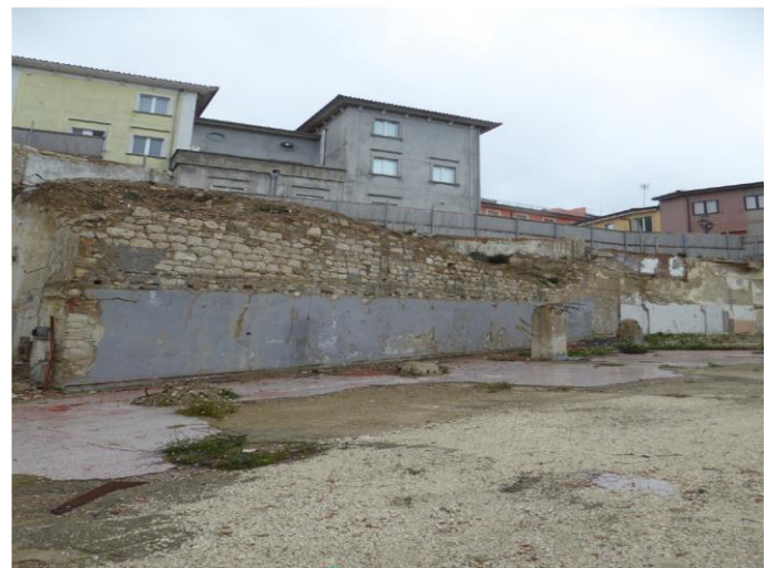
Figure 4. Building site, the altimetric gap: view from the existing ground level (almost other 3 m of excavation are expected)
