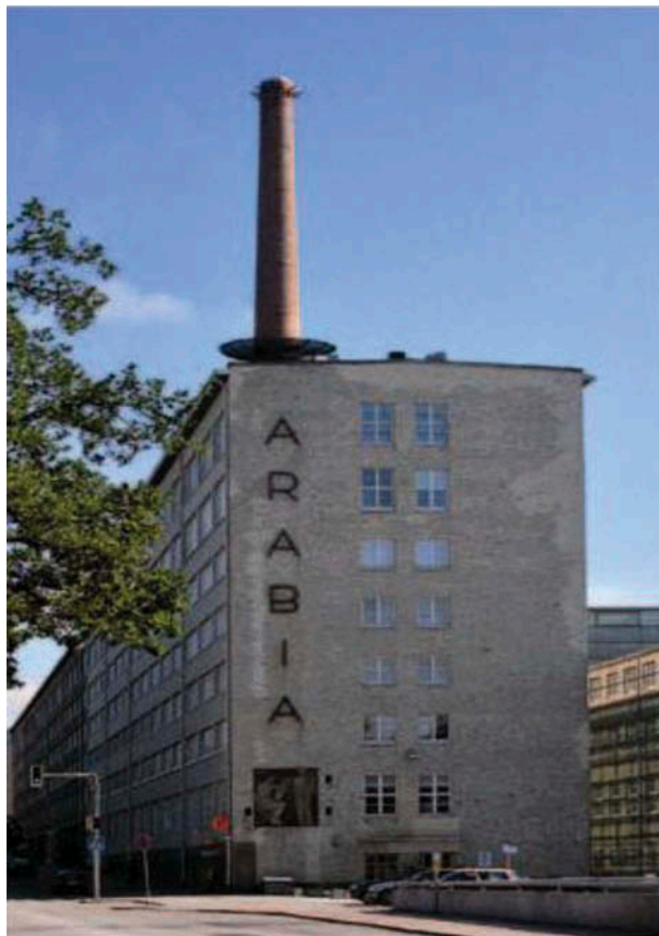
Figure 2. The Arabian old factory chimney (from: http://www.arabianranta.fi ).
