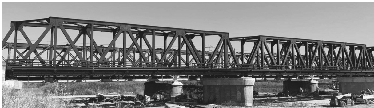
Figure 3. A typical steel railway bridge of Italian Railway infrastructure.
