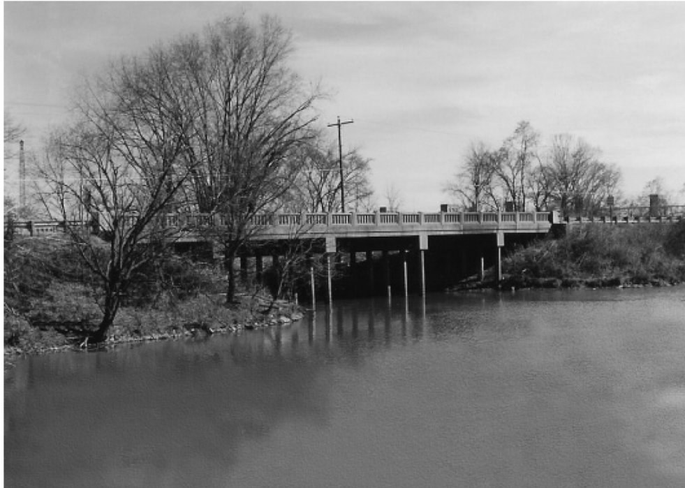
Figure 1.2: Teens Run Bridge, near Eureka, Ohio, 1938. It is thought to be the first integral bridge constructed in the United States and possibly in the world. (Burke 2009)
