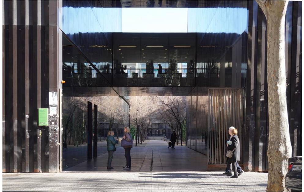
Figure 2. RCR architects, Sant Antoni – Joan Oliver Library, Barcelona 2007. The entrance from Calle Conde Borrell
