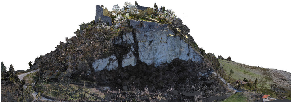
Fig. 6- Integrated point cloud of the entire Castle-Hill system (graphic elaboration by the authors)
