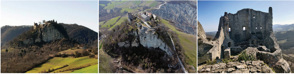
Fig. 1 - Images of the Castle. From left: bottom view of the sandstone hill, RPAS view of the system, detail of the most preserved portion of the area (photos by the authors)
