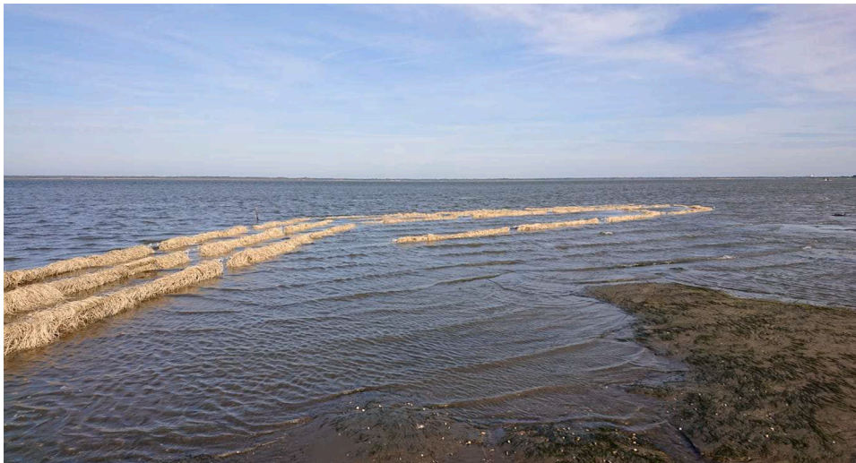
Fig. 2. Illustration of hydro-morphodynamic damping from La Roselière, a hybrid grey infrastructure/NbS approach for coastal restoration developed by EGIS-Seaboost and deployed at Arcachon bay, south Atlantic coast of France (credit: A. Musnier, Seaboost).
