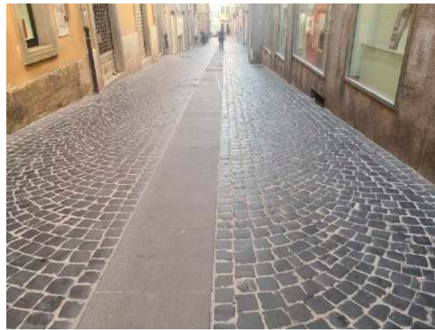
Figure 10. Typical Sampietrini Pavement in the city of Velletri.
