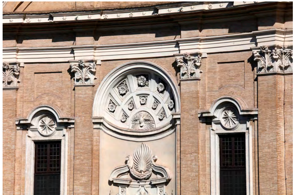
Figure 7. Francesco Borromini, Casa dei Filippini in Rome, detail of the deformations of the upper part of the niche (photo by M. Carpiceci).
