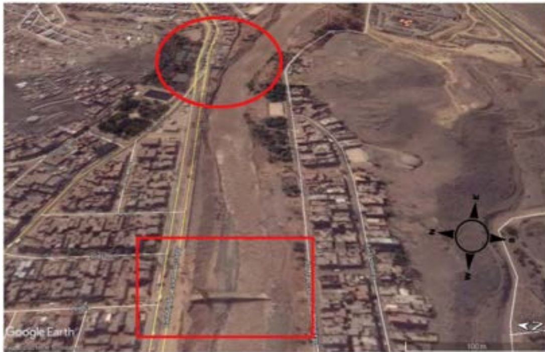
Figure 12. Google Earth optical view of the riverbank (red circle, see Figure 10) and the Talavera Bridge (red square, see Figure 11) collapses on 26/03/2017.
