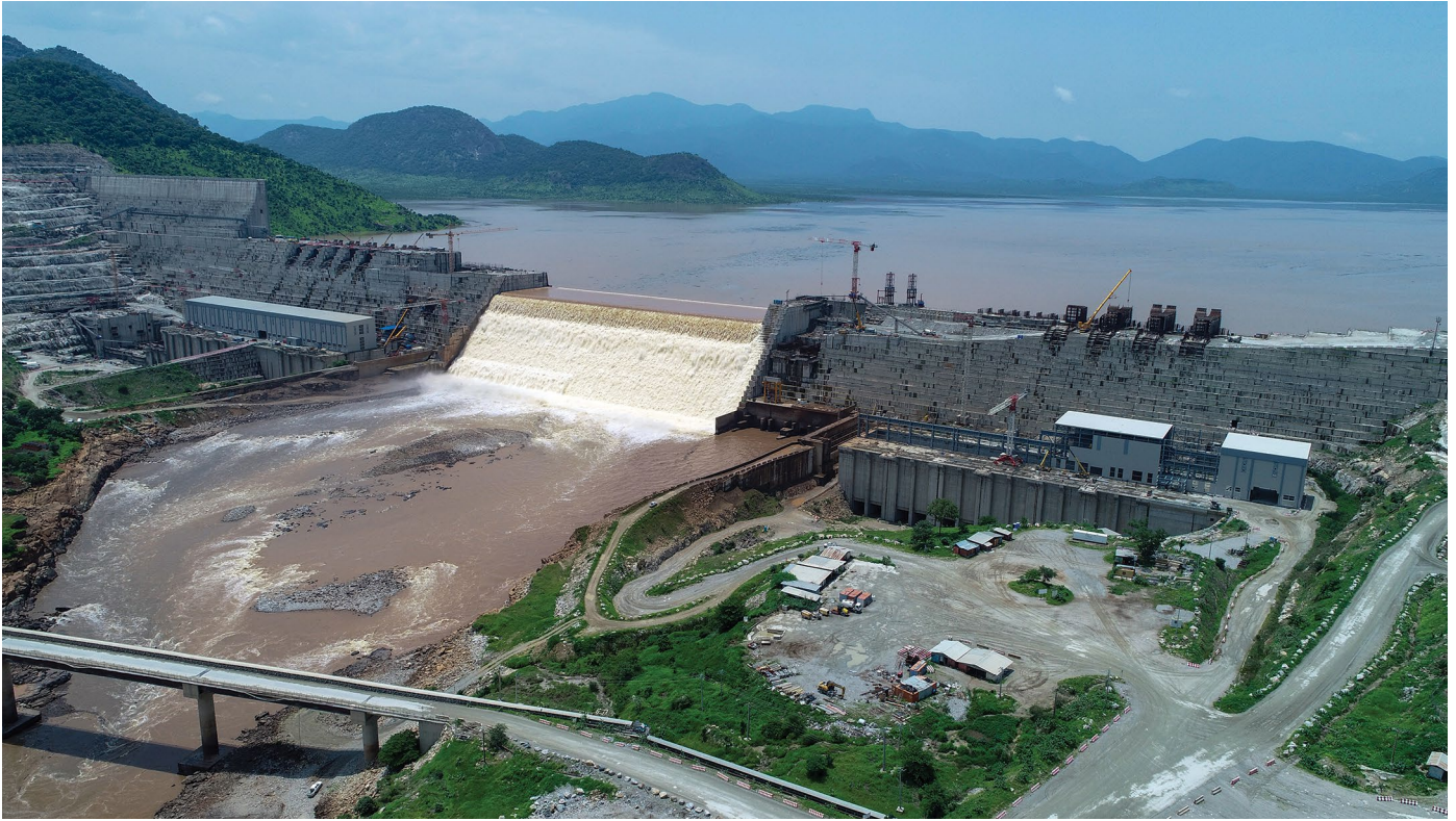
A view of the Grand Ethiopian Renaissance Dam on the Blue Nile in Ethiopia. Ethiopia has started generating electricity from the giant Renaissance Dam, and its Prime Minister Abiy Ahmed congratulated the people on the “birth of a new era” of development.
