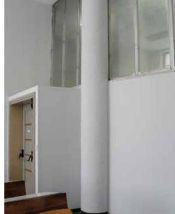
Figure 22 - One of the columns incorporated in the walls added to fragment the drawing rooms at the first level of the curved wings (© Salvo 2021)
