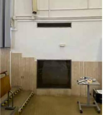
Today the opening system of these windows cannot be operated easily as they can be opened only from the outside, accessing on the roof terrace; in addition, recent maintenance works have laid varnish on hinges and fixtures, which are now stuck in the closed posi-
