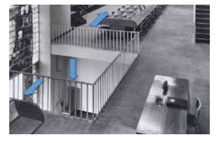
Figure 14 - Detail of air flow in the library reading hall in the original situation (ACS\_pht\_30)
