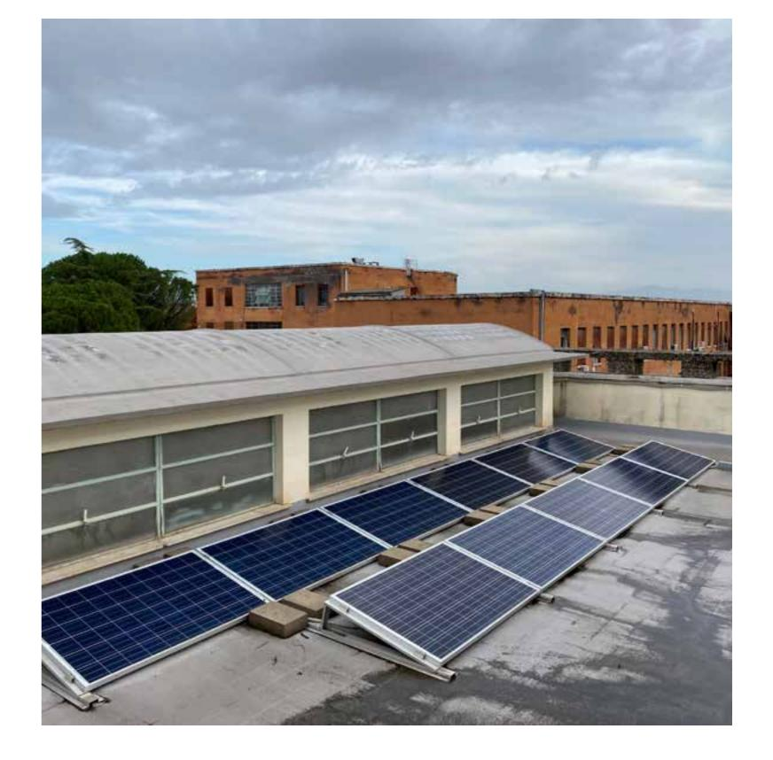
Figure 8 - The PV system on the rooftop of the front building (© Salvo 2021)
