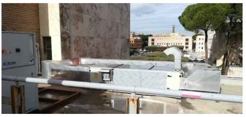
Figure 11 a/b - a) View of the refrigeration unit with Air Handling Unit dedicated to the library rooms placed on the rooftops (© Salvo 2021) and detail (b) (© Mancini 2020)
