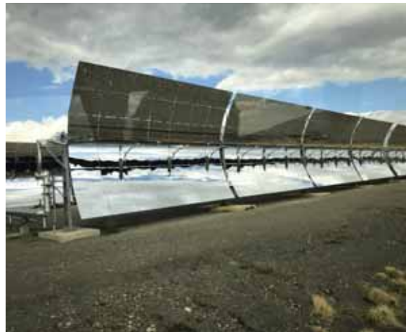
Figure 3. Parabolic trough collectors (credits © H2020 European Nexttower Project).
