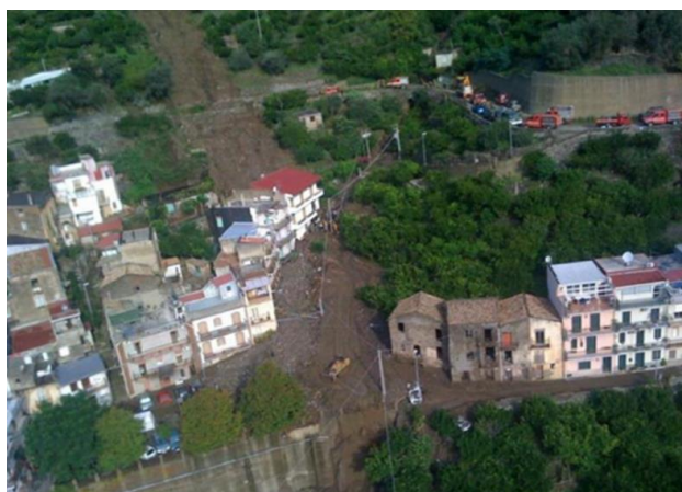
Figure 4. Effects of the debris flow in the Altolia village.
