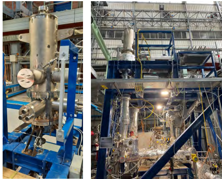
Figure 11. Pictures of PAV-ONE mock-up and its installation in the TRIEX-II facility.
