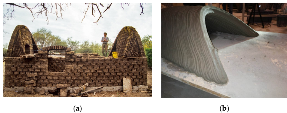
Figure 4. The Nubian vault: (a) Traditional Nubian vault construction technique using raw earth bricks [27]; (b) Prototype of a vault 3D-printed with 40^\circ inclined layers without supports [28].
