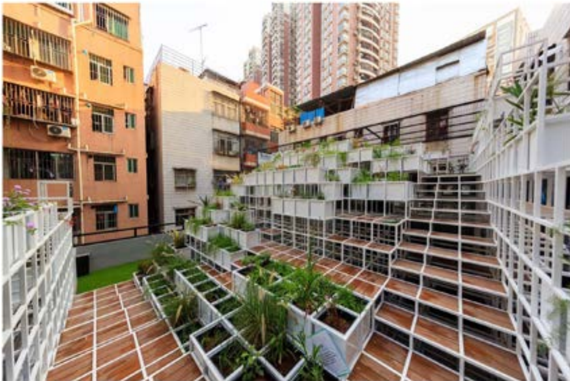
Figure 3. Green Cloud. Steel structures to contain the different plant species. The Nature Conservancy.
