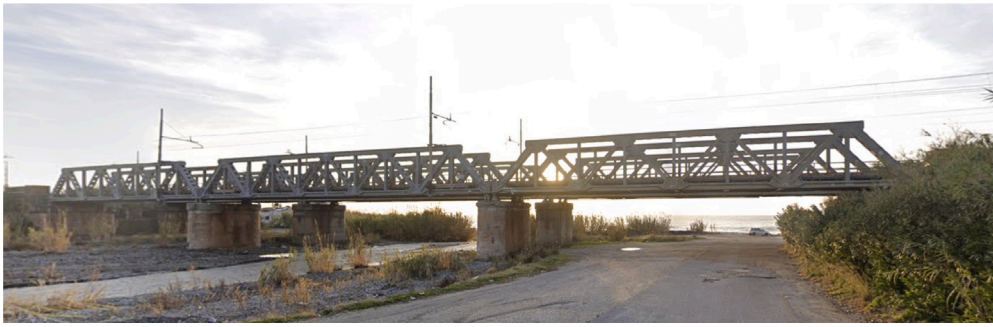
Fig. 21. Overview of steel railway bridge investigated in the present work.
