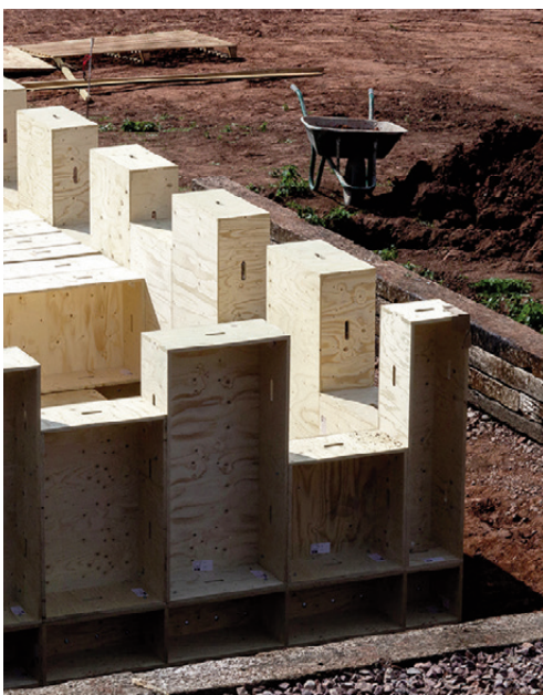
Fig. 10 | A wall of the Mass Bespoke construction system (source: massbespoke.com).
