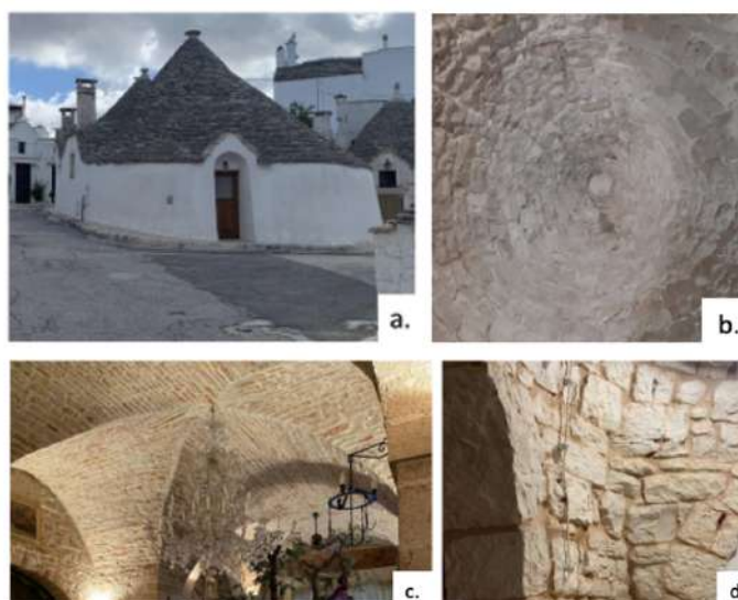
Figure 4. (a) Roughly circular plan of the modular construction unit of the trullo. (b) Interior view of the trullo pseudo-dome that forms the roof. (c) View from the inside of the juxtaposition of several modules and the detail of the junction area. (d) The thickness of dry-stone masonry on the perimeter of the trullo (photos a, c, and d by Alfonso A. Mascitelli; photo b by Giada Costa).
