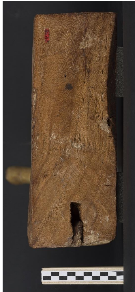
Fig. 52 – Bearer C, non-functional tenon-mortise joint on basement
