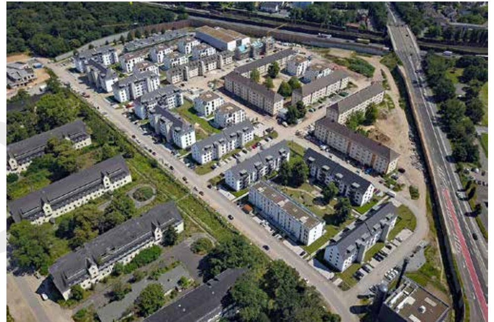
Fig. 2. An aerial view of Pioneer Park urban regeneration project (Hanau)
