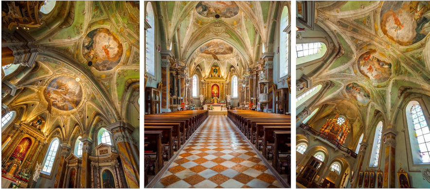
Fig. 1 The interior and the vault system of the church (photo by Andreas Manessinger). From left to right: the vaults over the chancel, the nave and the vaults with the counter façade and false dome
