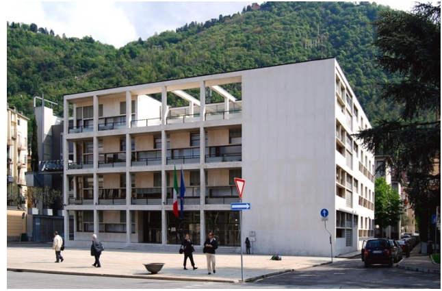
Figure 3. Giuseppe Terragni, Casa del Fascio , Como, 1932-1936 (source: https://www.archdaily.com/312877/ad-classics-casa-del-fascio-giuseppe-terragni ).
