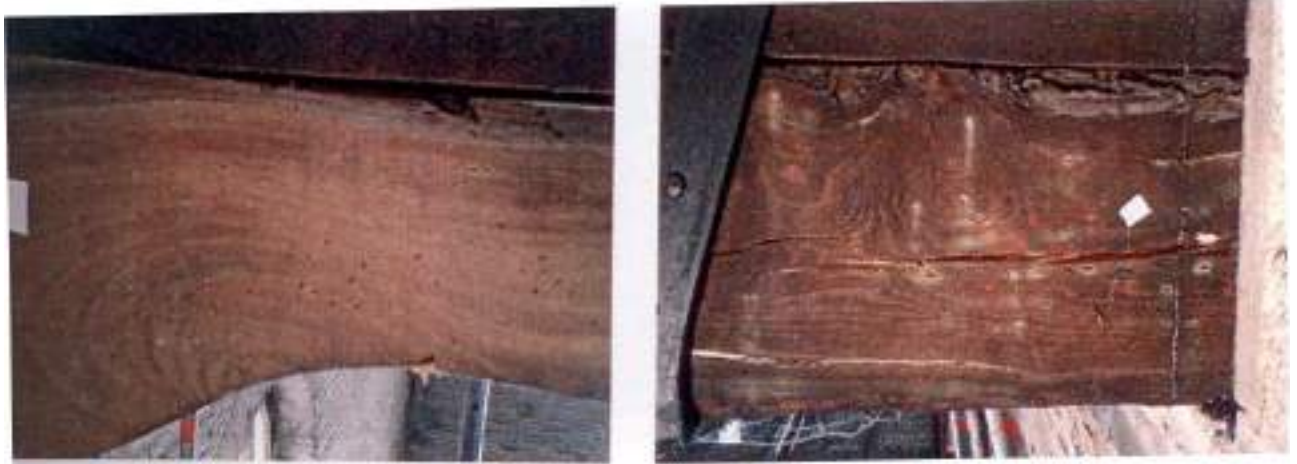
Fig. 59. Analysis of specific damages. Attack of anabids xylophagous (left). Attack of cerambicides xylophagous (right). From P. Rocchi, C. Piccirilli, Manuale della Diagnostica , Edizioni Kappa, Roma 1999.
