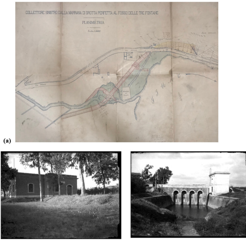
Figure 4. (a) Collector sewer path general plan between the Marana di Grotta Perfetta and the Tre Fontane ditch, 1882; (b) picture of the Collector sewer point of disposal n. 7 and of the sewer crossing of the Marana watercourse, 1925–27 (courtesy of Rome State Archive, Ufficio Speciale per il Tevere e l'Agro Romano collection).
