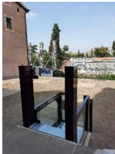
Fig. 32. New mechanical platform in Imperial Fora, Rome, Italy.
