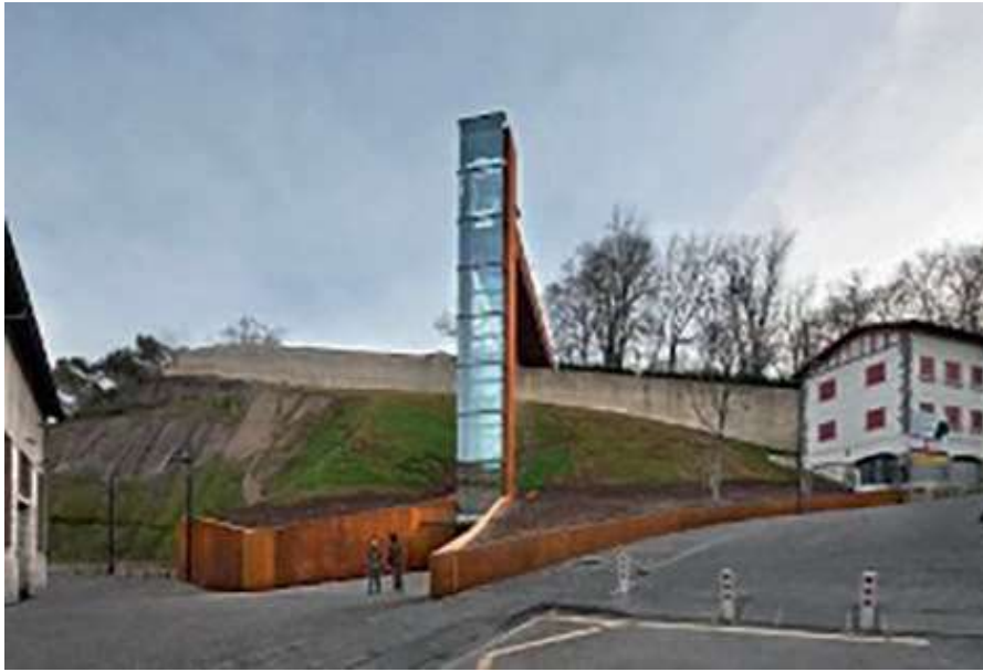
Fig. 5. New lift in Pamplona.
