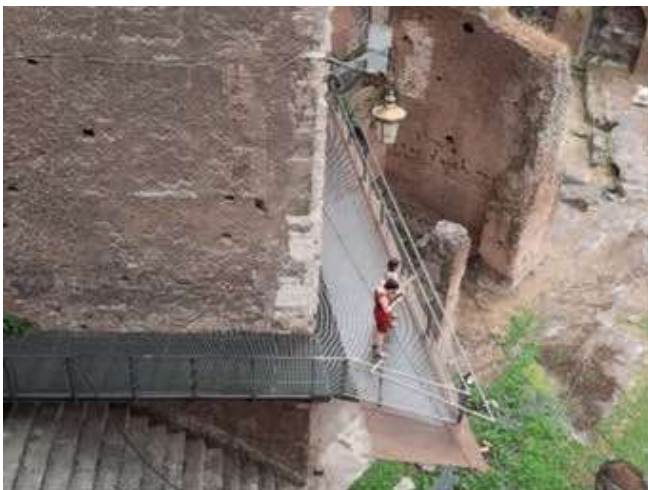
Fig. 37. Footbridge in Mercati di Traiano, Rome, Italy.
