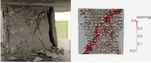
Figure 12: Cubic specimens: experimental and numerical crack pattern at failure
