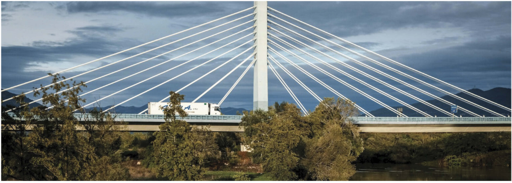
Figure 1. Overview of cable-stayed bridge over Garigliano river.
