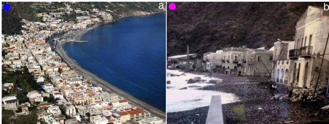
Figure 9. (a) Image of Canneto bay, with the central pier intercepting the littoral drift from N to S. The submerged breakwaters are also visible in the coastal area, south of the pier; (b) image of the southernmost beach of Canneto during a storm. Location of pictures is in Figure 1 through respective colored dots.
